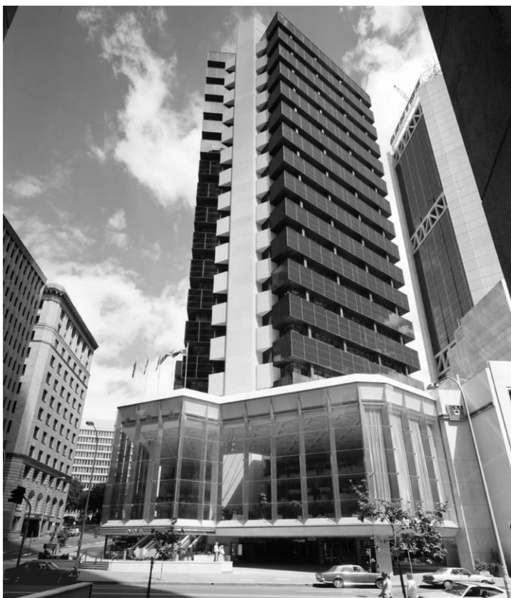
Figure 8: The original podium shortly after its completion in circa 1980
