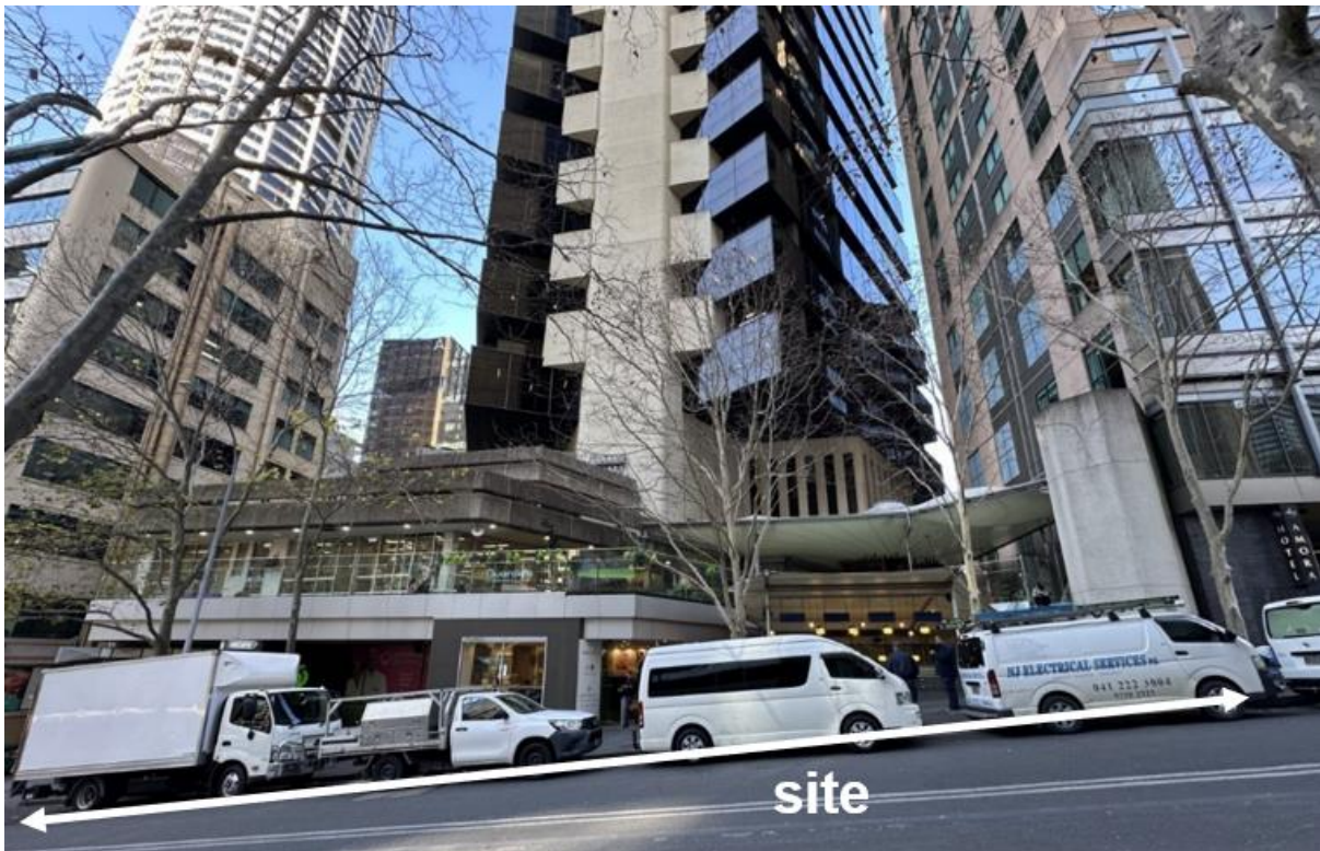
Figure 6: Site viewed from Jamison Street
