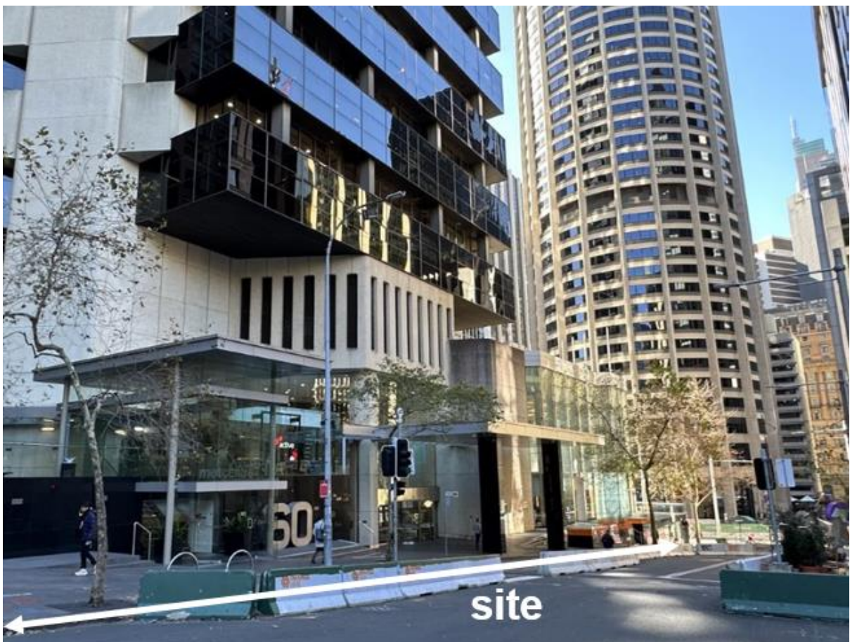
Figure 4: Site viewed from Margaret Street
